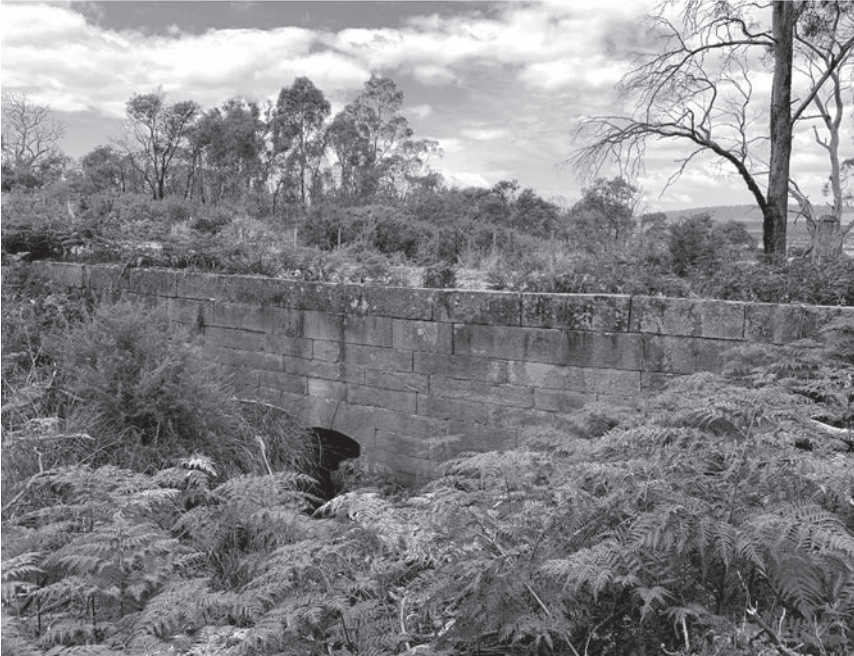
Upstream side of the culvert (Malcolm Ward)
